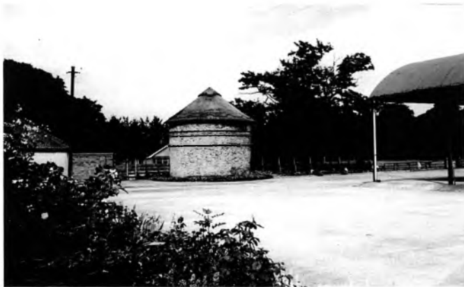
The dovecote at Thoroton
