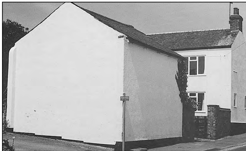
The building as it is today, a domestic garage. The only evidence of its former use is that the doorstep remains!
