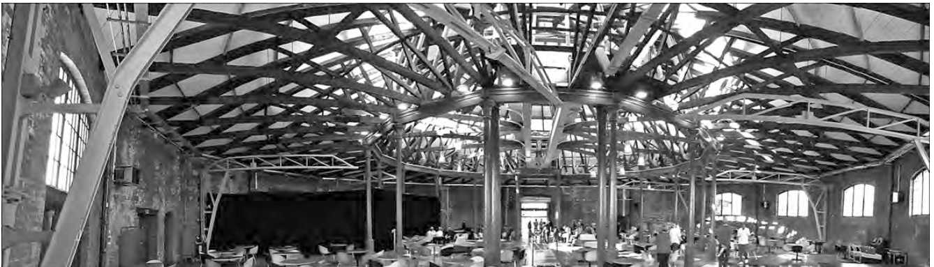
Panoramic photograph of the Roundhouse. Photo: Howard Fisher
