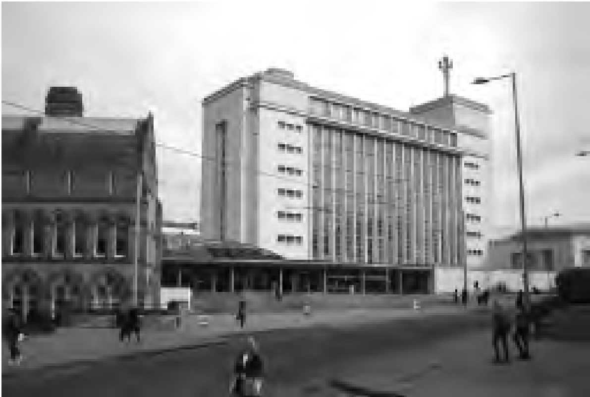
Nottingham Trent University's Newton Building (Photo: George Murfet)
