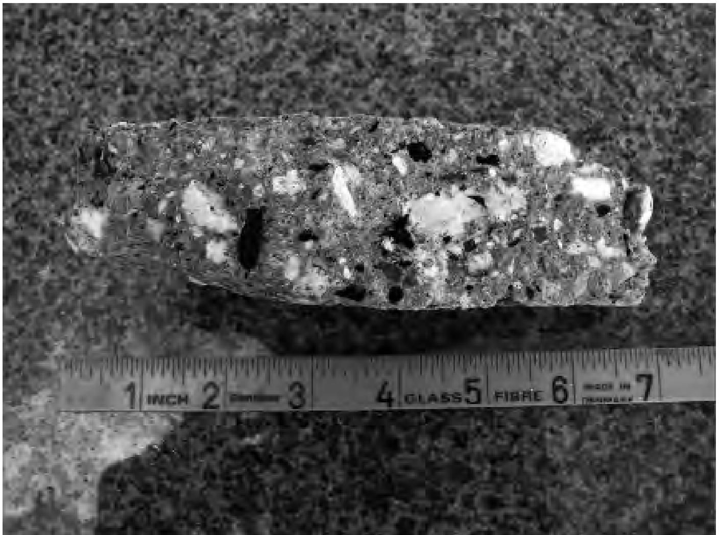
A piece of the floor. Photo supplied by Peter Allen - original in colour.
