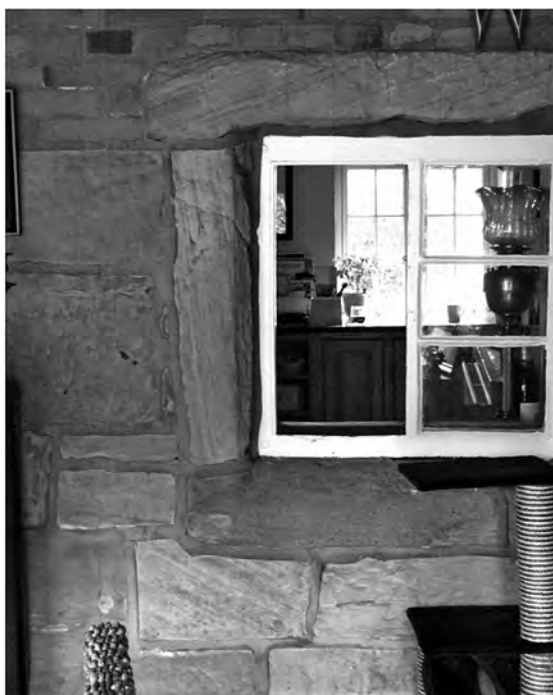
Original stonework inside a cottage on Rectory Avenue
