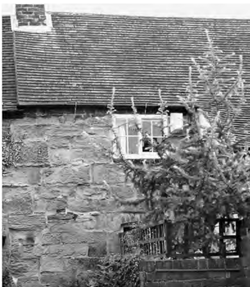
Fine ashlar stone blocks on a rear wall
