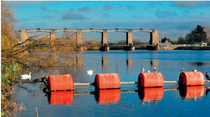
Holme Sluices, Colwick
